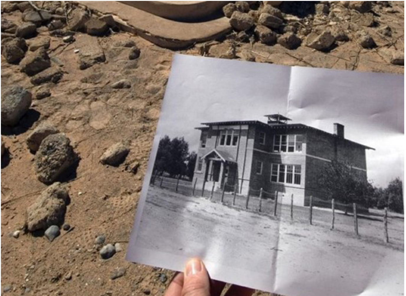
Figure 22. The old St. Thomas School House near the remnant steps that have re-emerged as the lake water levels have dropped. (Photo credit NPS)
